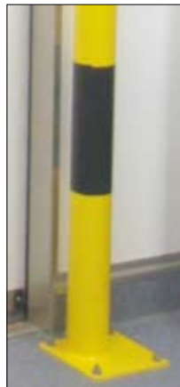
Impact protection post
