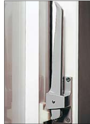
Heavy-duty opening latch for single leaf door; adjoining picture shows bolt mechanism for double leaf door.
